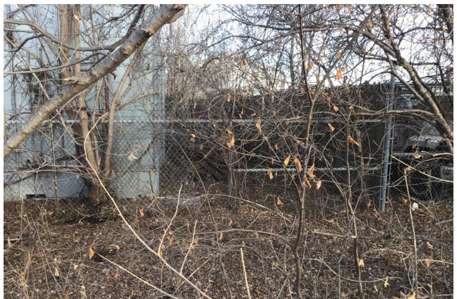
Figure 1: The current chain link fence, viewed from BNSF right-of-way on February 1, 2024. The fence has been cut and repaired (center of the image). Easily-climbable vegetation grows through the fence. The fence is shorter than the adjacent southern property's fencing.
